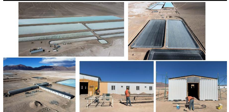
Figure 20: Stage 2 in Construction: 2,000tpa Operation
