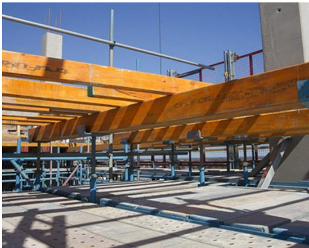
Figure 12: BRI Formwork – LVL
